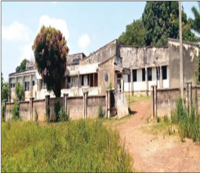
Figure 3. Okenya Health Centre in old NRC Building, Kogi State.
